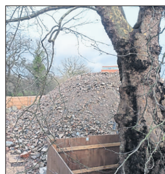
The demolition under way
